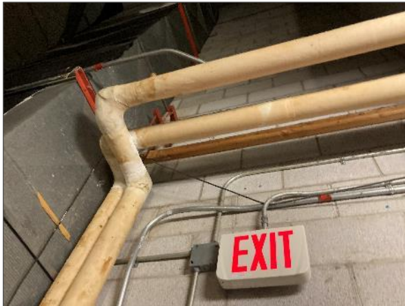
Asbestos-containing paring cement insulation on pipe elbows.
