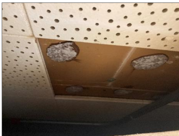
Non-asbestos acoustic ceiling tile mastic.
