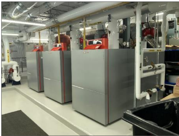
Non-asbestos insulated boilers.
