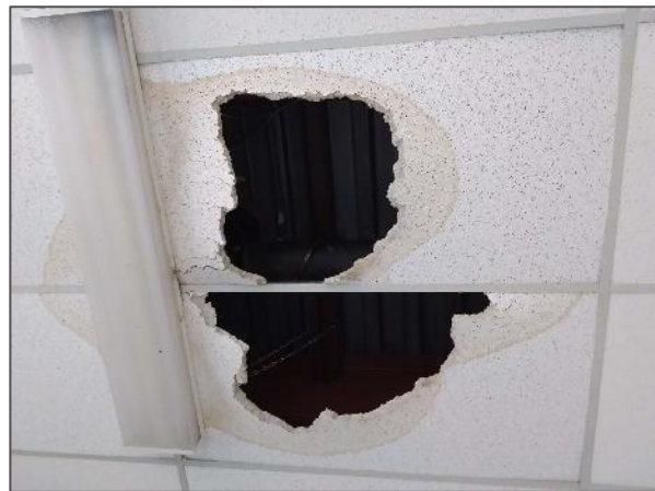
Water staining present on acoustic ceiling tiles in the Classroom (Location 2160).
