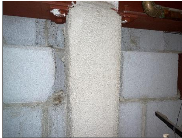
Non-asbestos sprayed fireproofing present on the steel column.
