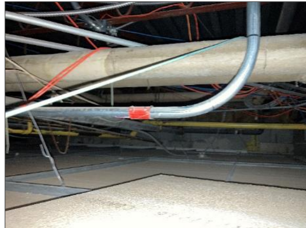
Asbestos-containing Caposite insulation.
