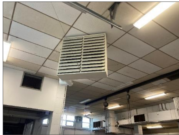
Non-asbestos fibreglass insulated suspended unit heater.
