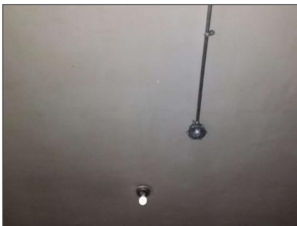
Asbestos-containing plaster base coat in Building Phase D.
