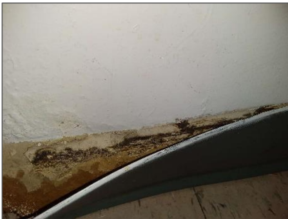
Mould growth and water staining present on the drywall wall in the Washroom (Location 1012).
