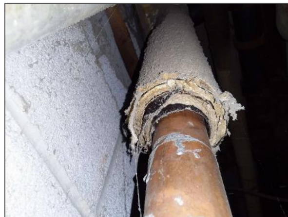
Non-asbestos sweatwrap insulation.
