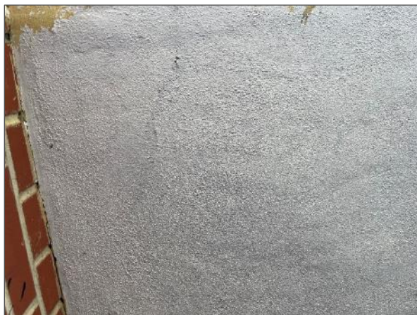
Asbestos-containing textured plaster on exterior canopy of Building Phase D.
